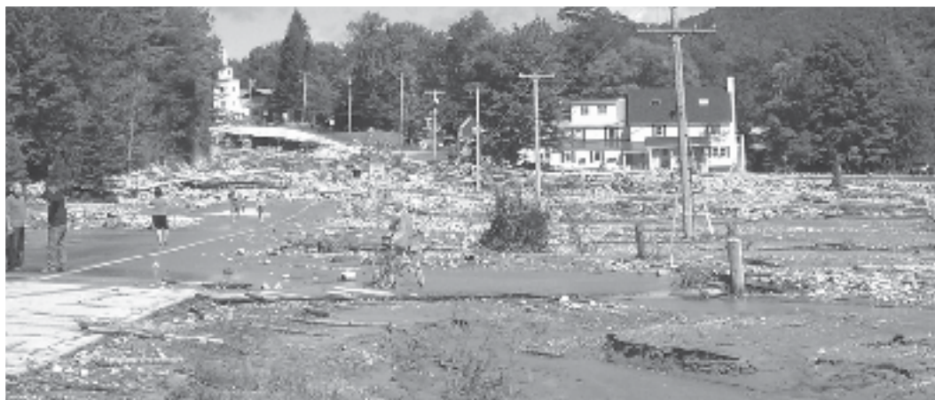
Devastating damage to Route 4, Killington
